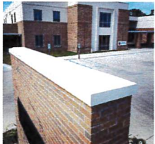
BRICK WALL WITH WHITE CONCRETE CAP
