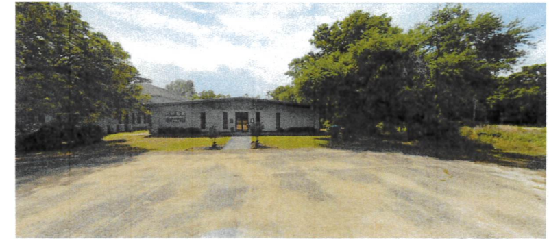
East Elevation - Existing Building
