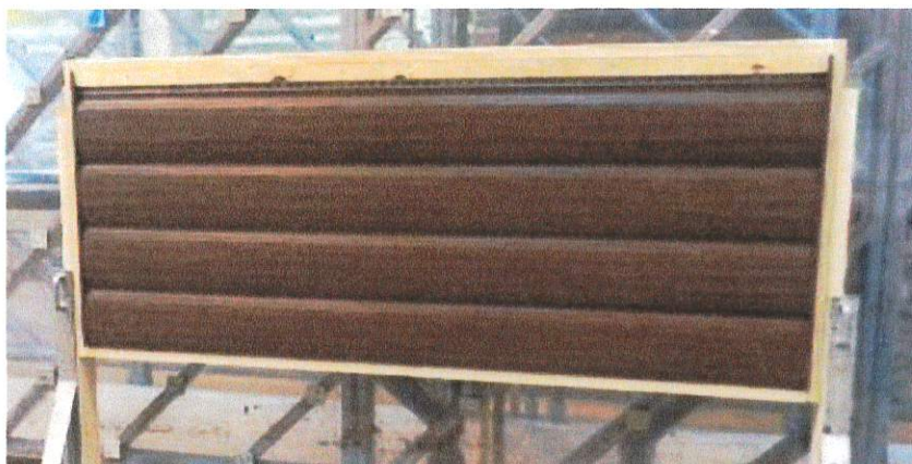
Photo No. 1 TruLog, Steel Siding, Single Specimen Install
