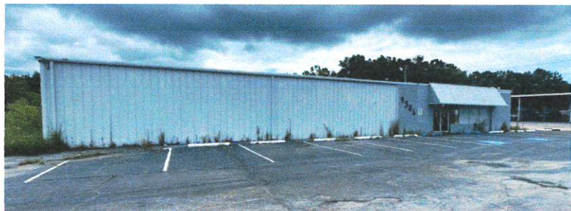
The building located on the property is approximately 8,600 square feet. It is a metal building that includes showroom and warehouse space.
