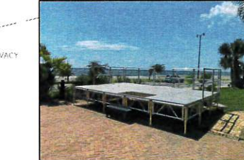
EXISTING STAGE WHERE PROPOSED PAD IS TO BE LOCATED.
