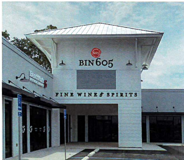
North Side Tower
