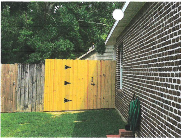
Above: Side fence w/ Gate (left)
