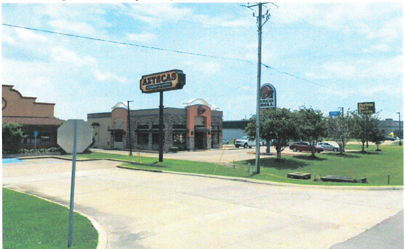
EXHIBIT L. Hwy 49 - Azteca's, Taco Bell 2019 - each replaced logo signs
