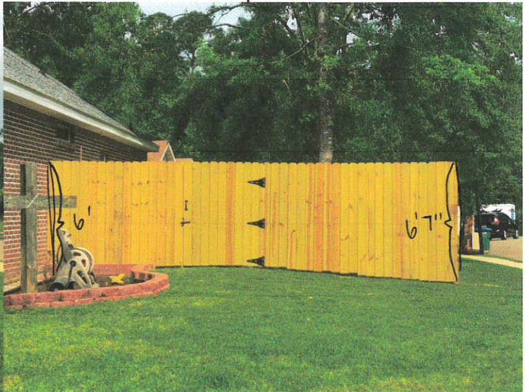
Above: closer view of side fence (right)
