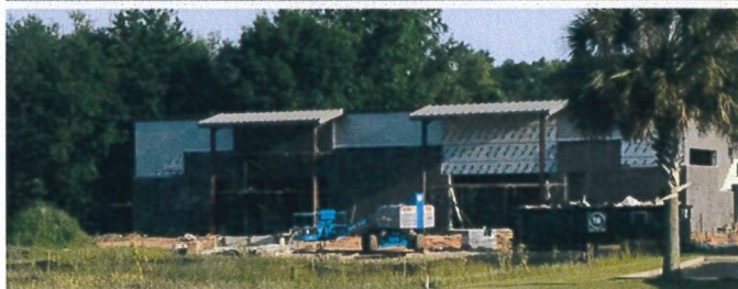
Commercial development continues along the corridor, and currently three sites within the immediate area are under construction. This supports both the change in character and public need for more sites.
