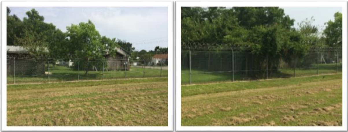
Figure 57 Trees overhanging the NCBC Gulfport fenceline
