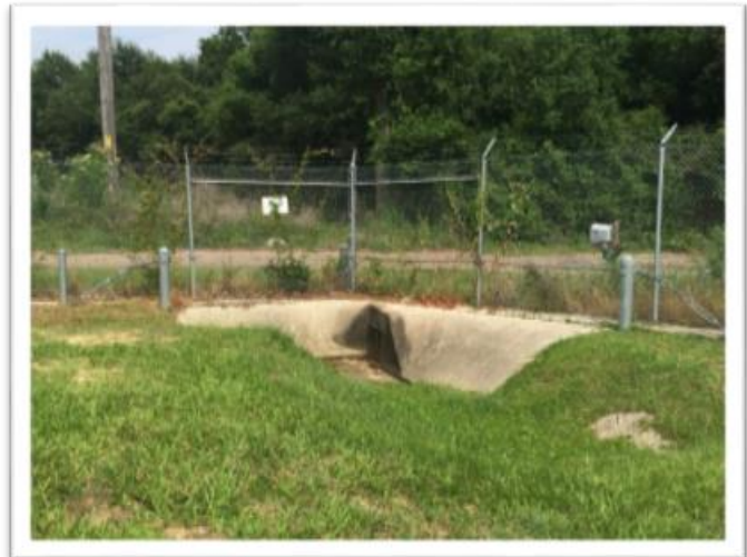
Figure 53 Drainage canal located within NCBC Gulfport
