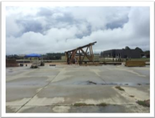
Figure 25 Construction training exercises
